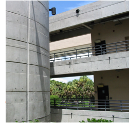
LOOKING NORTH-EAST FROM ATRIUM 02:45 PM 25 JUL 02
