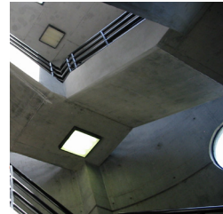
LOOKING UP INSIDE SILO STAIR 03:50 PM 25 JUL 02
